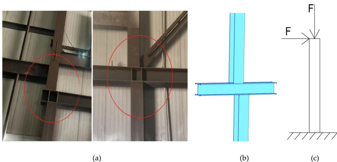
Figure 2. Column connection eccentricity: (a) actual conditions on site, (b) FE model and (c) analysis scheme
