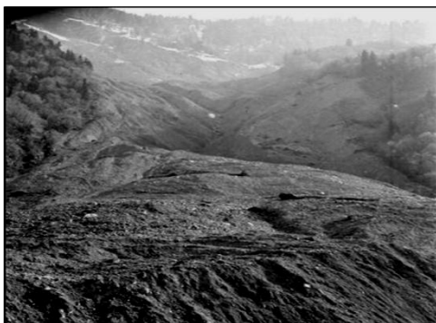
Figure 3: Slopes affected by landslides 1989 affected by landslides
