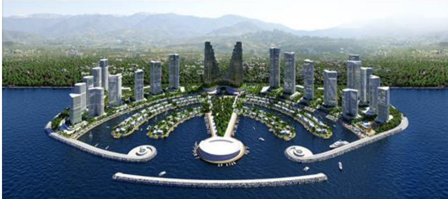
Figure 1: Completed "Ambassador Batumi Island"
