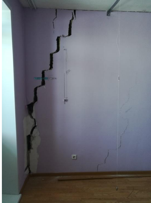
Figure 1: deformation of a building in arctic conditions due to uneven settlement of the "soil-building" system
