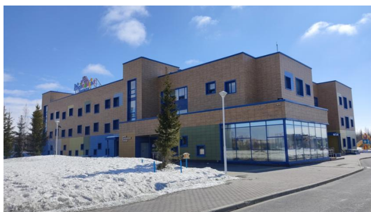
Figure 2: Kindergarten Building Tested Using the Dynamic-Geophysical Method.
