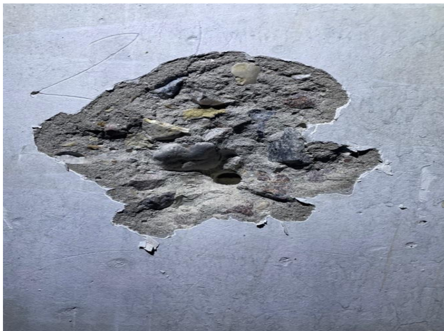
Picture 3: Breaking out of concrete during a shear test
